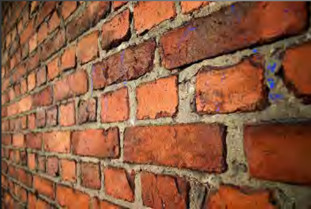
An old brick wall in English bond laid with alternating courses of headers and stretchers
